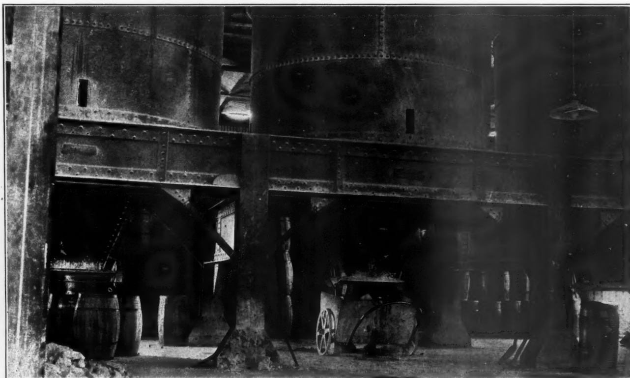
Lime Drawing Floor. Note Steel Construction
